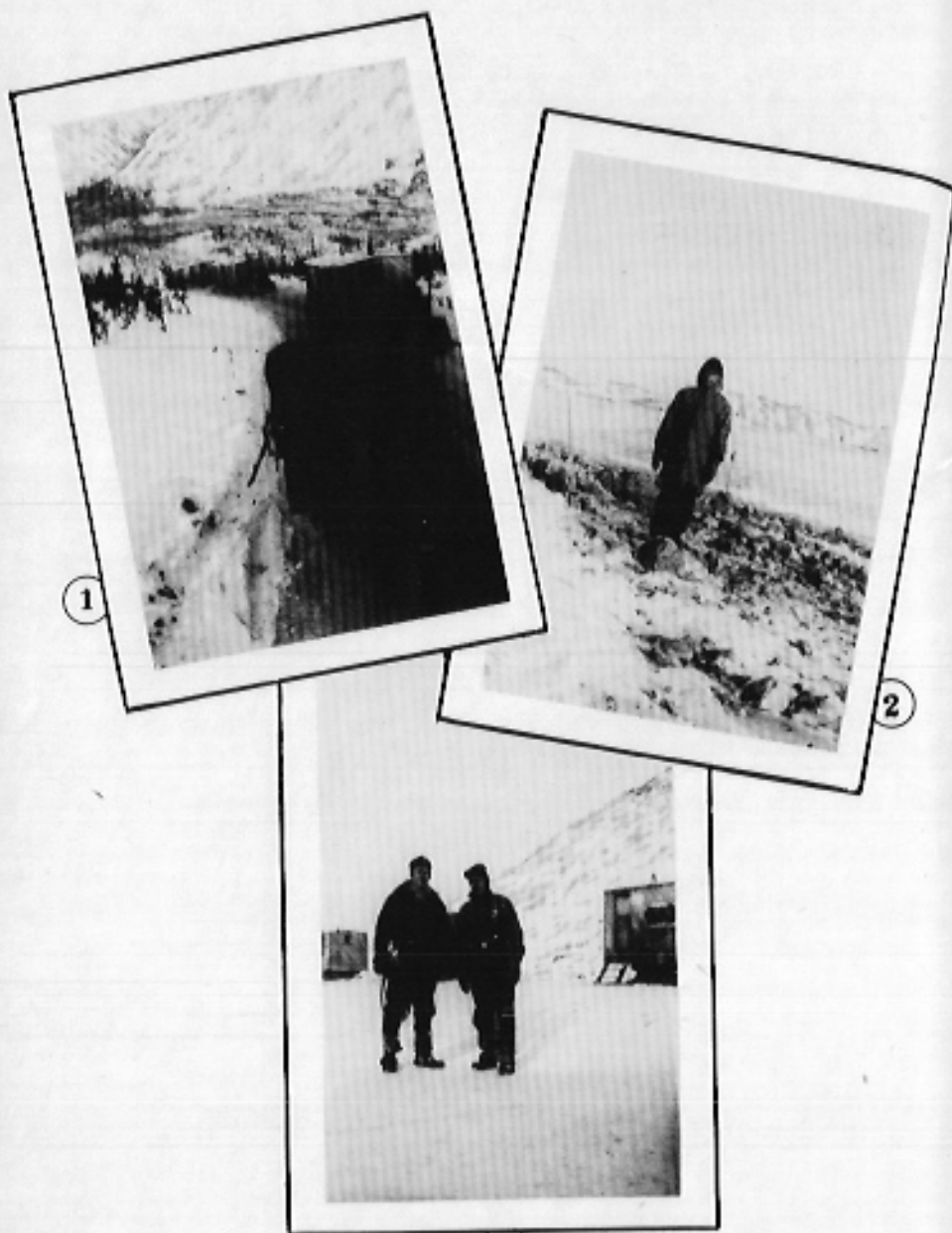
1—"Moving Camp near Camp 95." 2—"A picture of one of my co-workers. The work of the 'electrician grounded' (of whom I was one the winter of 1945-44) is primarily to dig holes 3—6 feet deep for telephone poles. Iron bars—such as the one standing in this hole—are cold on the hands at 35 degrees below." 3—"Mountains came down close both sides of Camp 111."
