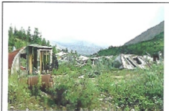
Road Maintenance Camp at 74.5
