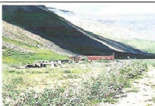
Pump Station at mile 108- halfway
