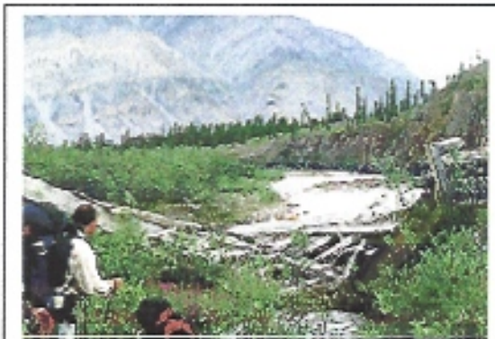
Broken bridge (Ekwi River)
